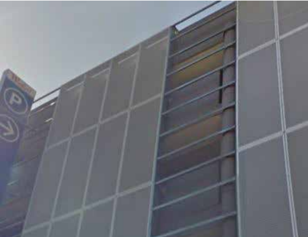
REF. IMAGE: EXISTING CARPARK PERFORATED FACADE AND SUBFRAME
